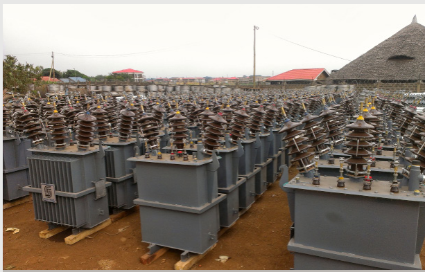
A line-up of batteries for rural electrification. Since joining the project, Carson has made several trips to the field to work with various stakeholders.
